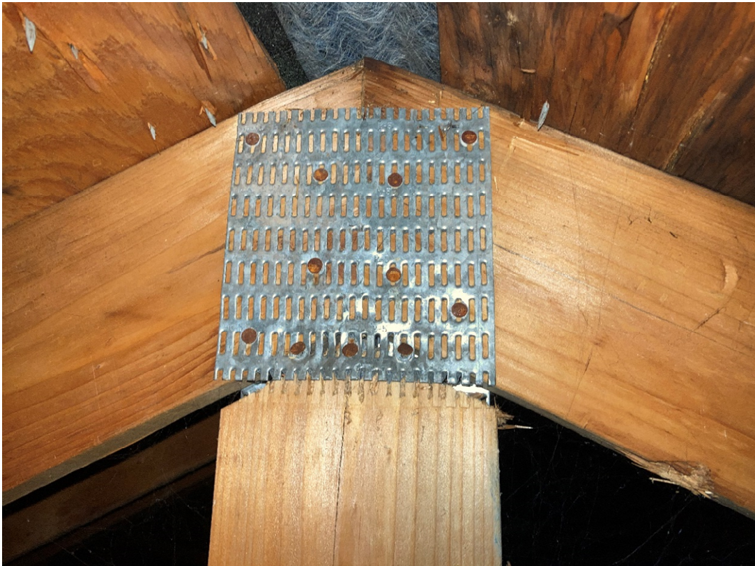
Figure 2 – Vertical Separation at Top of King Post
