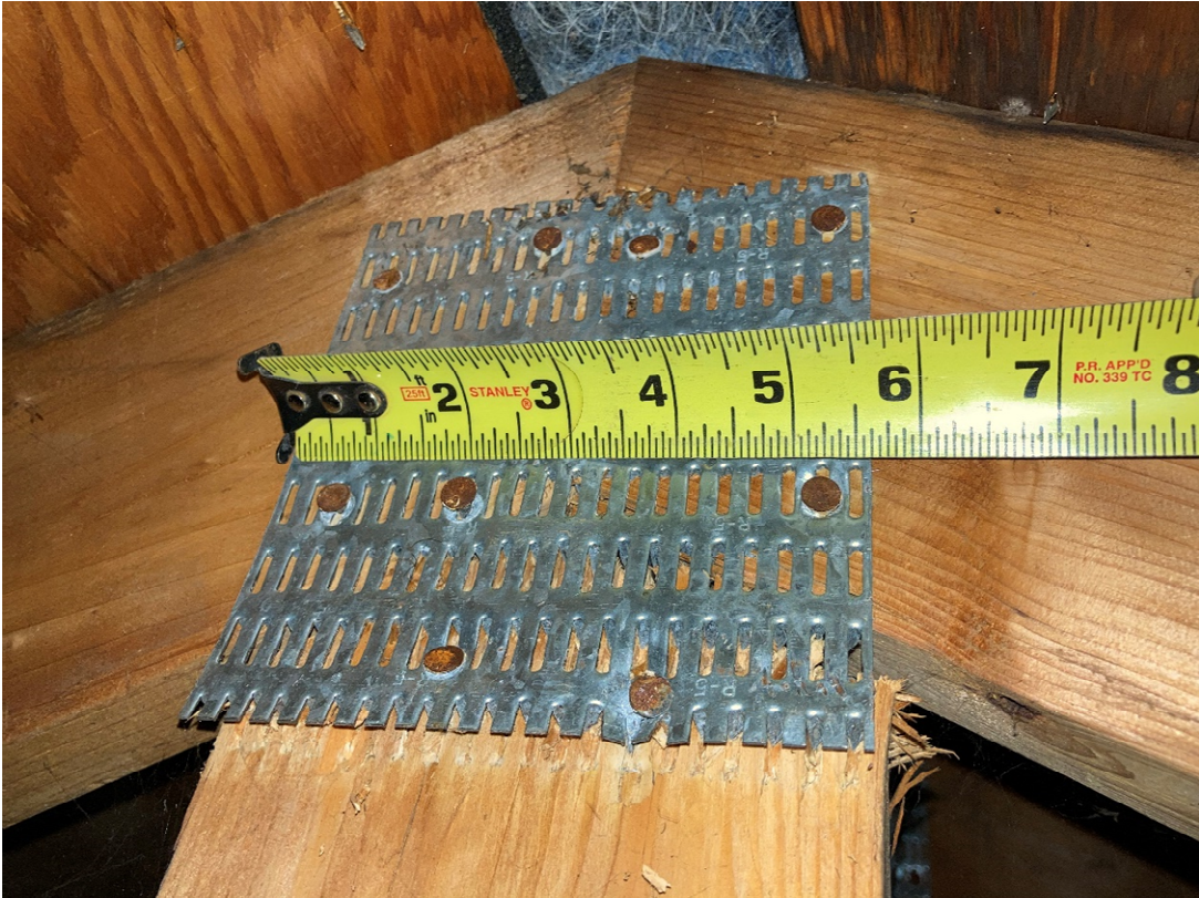
Figure 1 – King Post and Top Chord Truss Plate w/ Nails
