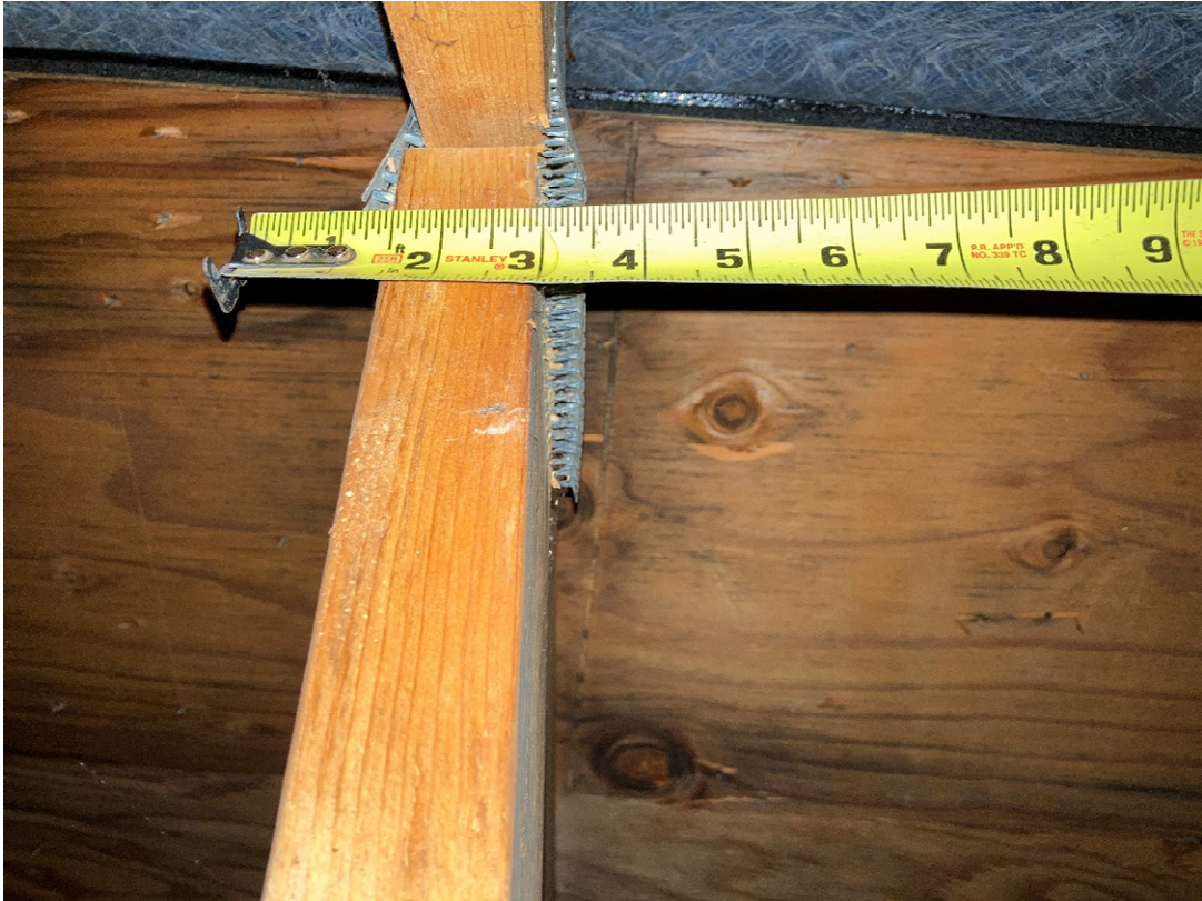
Figure 3 – Lateral Separation at Top of King Post
