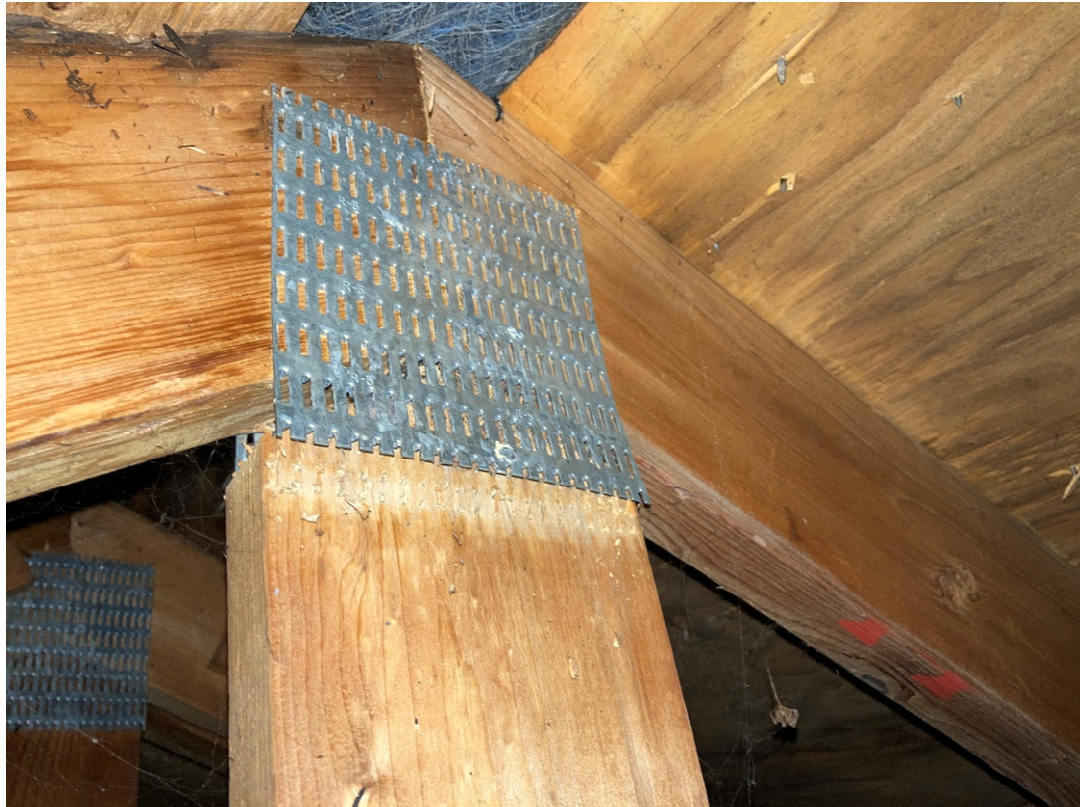
Figure 4 – Surficial Scraping from Plate Slippage
